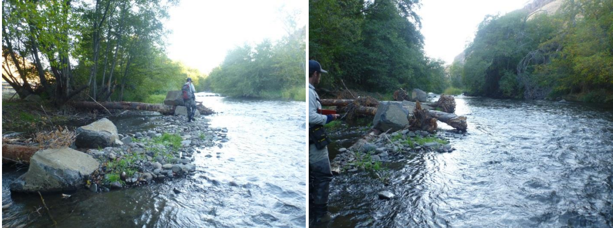
Figure 8. Photos showing two of eight LWD structures placed in Project Area 22.
