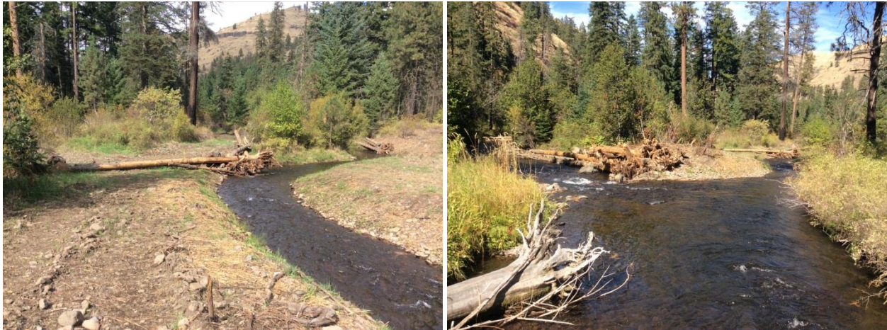
Figure 3. Restoration implemented in Project Area 1 included the creation of side channels and installation of LWD structures. Photos courtesy of the SRSRB.
