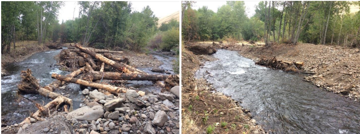
Figure 7. Restoration implemented in Project Area 15 included the installation of LWD structures (left photo) and the creation of new side channels (right photo). Photos courtesy of the SRSRB.
